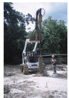
Borings should be drilled dry, and the depth at which groundwater is encountered should be recorded.
